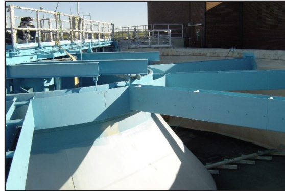
ARC S1PW blue being applied over ARC S1PW white.
